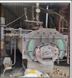
The boiler is used to provide steam in the various steps of processing such as boiling of rcn, steam borma etc. 18. Diesel Generator Set
