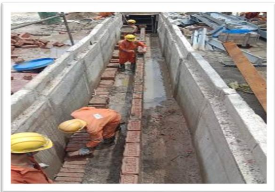
Electric Trench & Brick Work
